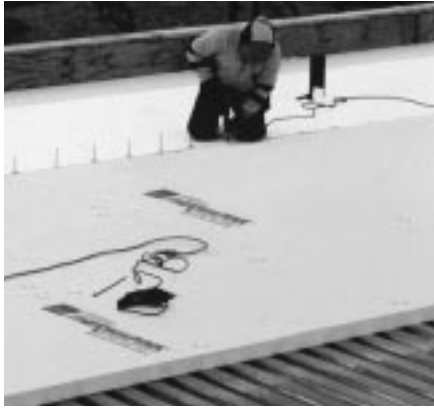
Exceptional moisture resistance and superior insulation for direct-to-deck application in steel deck roofing systems.
